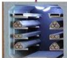
Comprehensive pipe gallery
