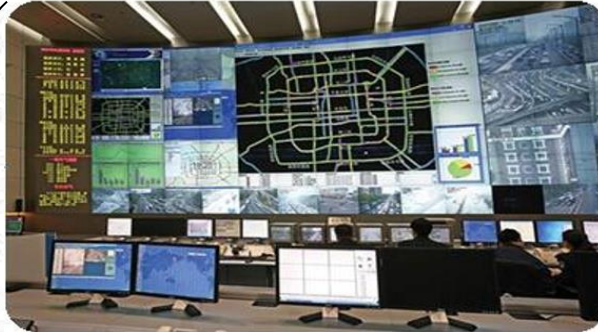
Command and control center
